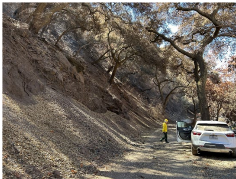
Picture 10: Large dry ravel cones forming along lower Trabuco road due to high rates of erosion (USDA FS).
