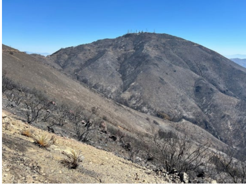
Picture 9: Santiago Peak with deep debris chutes visible dropping steeply away from the road (USDA FS).
