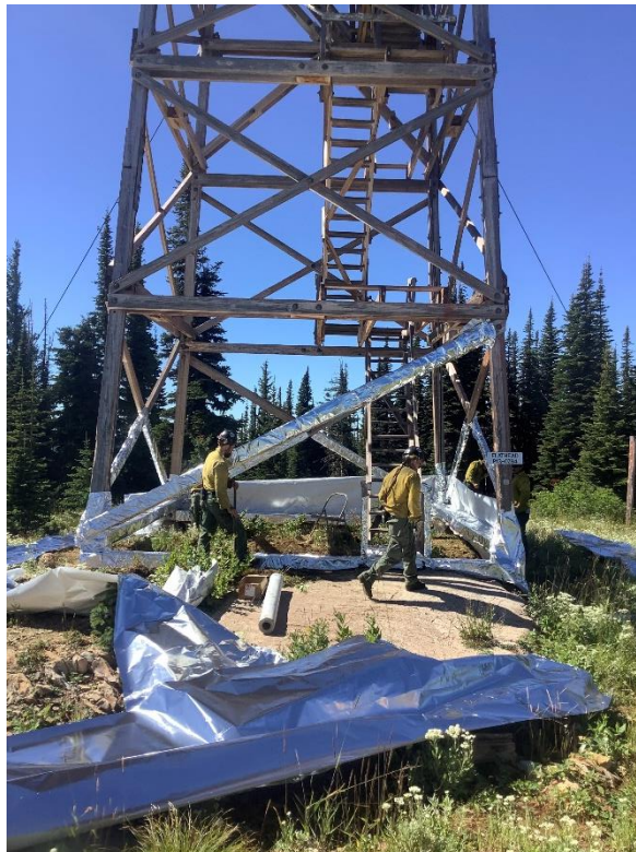
Photo of crews installing structure protection wrap on the Jocko Lookout. Photo Credit: Amy Helena, Division Supervisor.
