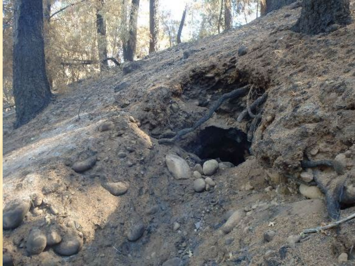
Cash Rock Adit Bat Culvert 1 before (left) and after (above) the fire.
