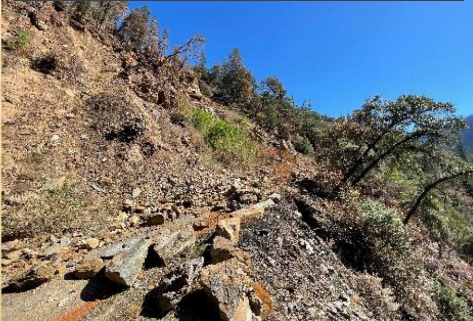
Existing landslides along Blacksmith Flat Road
