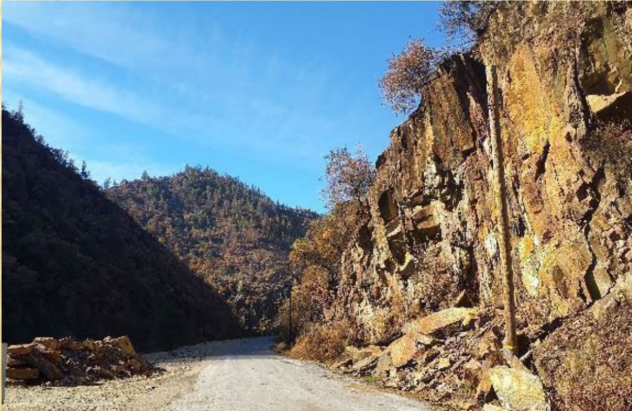
Rockfall on Blacksmith Flats Road from Mosquito Ridge Road to Ralston Reservoir
