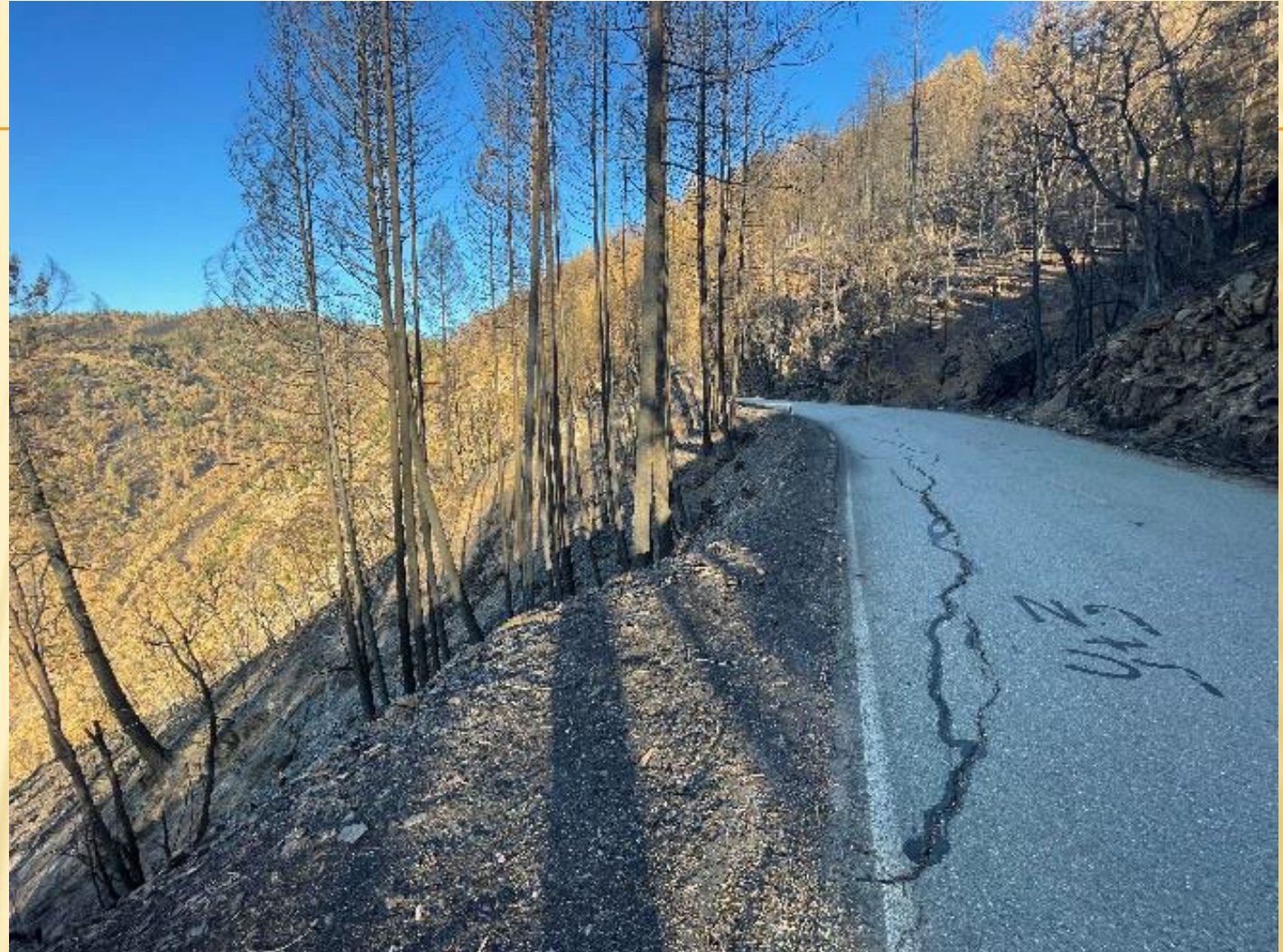
Mosquito Ridge Road on landslide-prone slopes
