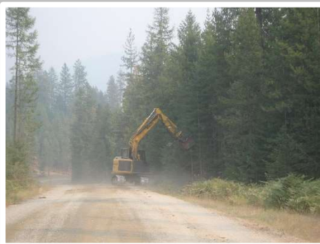
Heavy equipment works on suppression repair for the incident.
