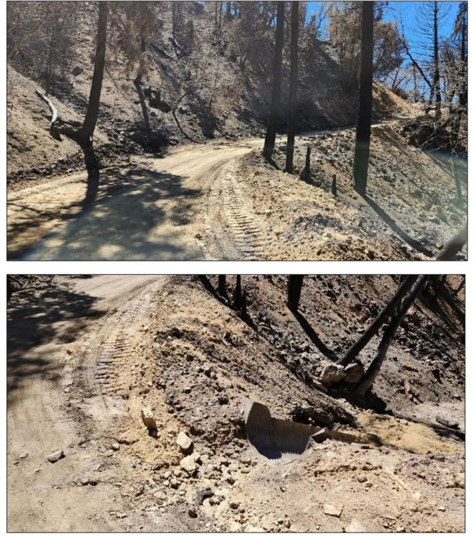
This photo shows a recent debris flow that initiated during the September 12, 2022, rainstorm event and deposited debris on the crossing of Forest Service Road 2N06 in the Radford burned area.
