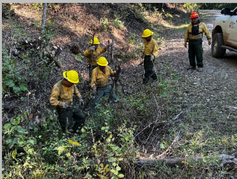
While an important firefighting tool, masticating can leave a buildup of vegetation in culverts. In the photo above, as part of suppression repair, firefighters are removing debris from a culvert. Photo taken from the Billiard Fire area.
