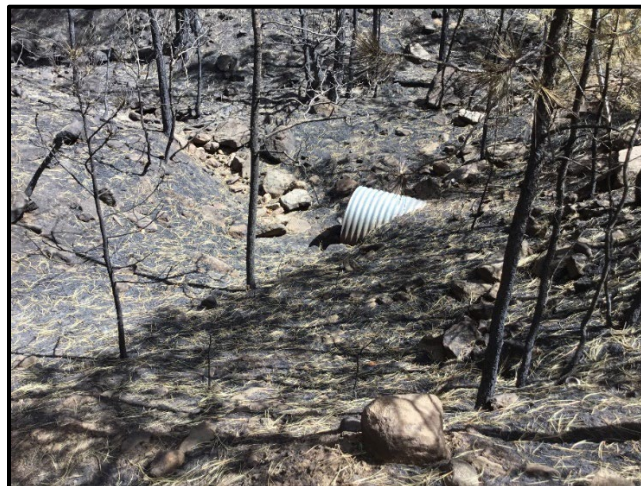
Figure 6. Burned area above culvert where increased erosion and sedimentation can plug culverts leading to a road being overtopped by flood waters.
