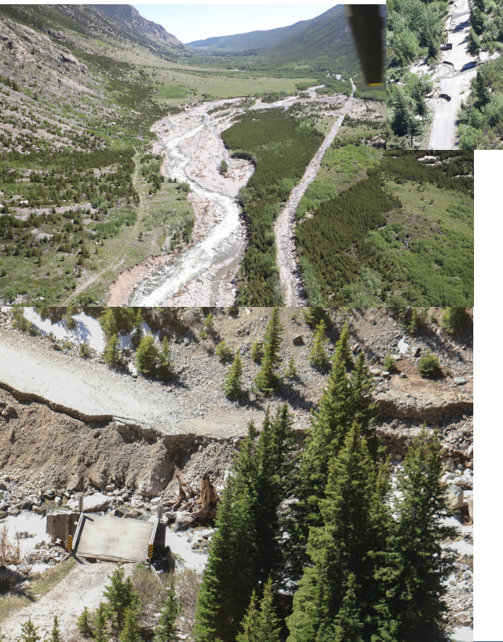
ABOVE: Yankee Jim Fishing Access Site and Vault Toilet, completely under water during extent of event, significant sediment deposit. Gardiner R.D. BELOW/INSET: East Rosebud Creek Drainage, extent of both road and drainage damage, Beartooth R.D. Custer Gallatin N.F. BOTTOM: Hellroaring Road and second bridge, washout, failure, damage.
