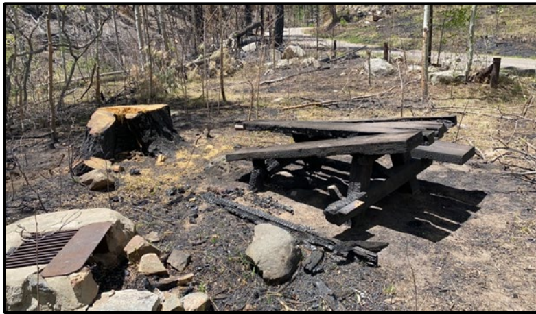
Figure 7. Burned recreation infrastructure at Big Pine Day use site.
