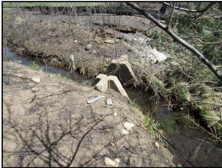
Figure 9. Historic concrete acequia headgate.
